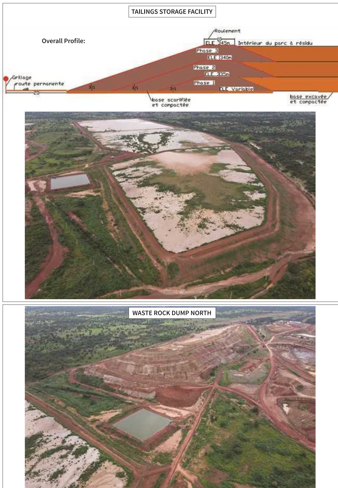
Figure 18.3: Profile and Photograph of the TSF and a Photograph of the WRD North
